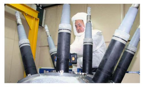
Any carcinogenic byproducts produced by electrical arcing are neutralised before the switchgear is released...
